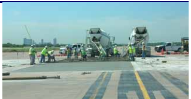
Meacham Runway 16-34 Repair
